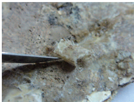
Removing adhesive from the surface
