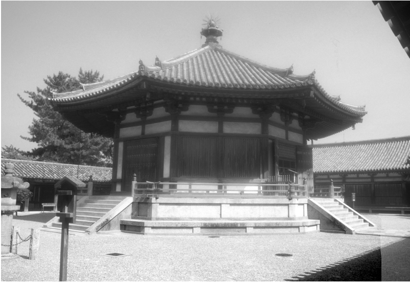
Figure 11. Yumedono of Horyuji, Nara Dated to 739. (Source: Puay-peng Ho.)
